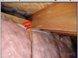
From the attic, the rafter located on the adjoining wall to the bedroom was notched beyond what would be typically expected. Rafters are key components of the roof system and need to be repaired to prevent framing movement and further damage. An engineer should be consulted for further evaluation to determine the significance and cause of the concern and outline necessary repairs to ensure the stability of the structure.
