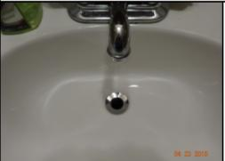
The plumbing system is in need of further evaluation and repair; the following concerns were noted at the time of the inspection: the stopper for the sink drain is missing. A licensed plumbing contractor should be consulted for complete evaluation and of the waste line systems to determine the general condition of the system and to make necessary repairs to ensure proper drainage and sanitary conditions.
