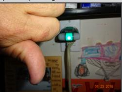
The GFCI in the garage did not trip when tested. This is a safety concern due to the potential exposure to water in the garage. A licensed electrician should be hired to fix the issue.
