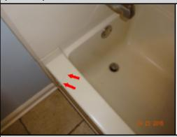
The fiberglass/acrylic tub has a crack in the surface. The chip could allow water to penetrate under the surface and possibility result in leaks. A specialist should be consulted to determine if the tub surface can be repaired.
