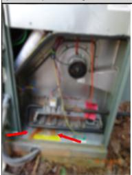
The area surrounding the gas furnace combustion/draft fan is rusted and deteriorated. Damage to the fan can result in improper operation of the combustion and or exhaust system. A HVAC contractor should be consulted for a complete evaluation and to make necessary repairs to ensure safe, reliable, and proper operation of the HVAC system. The arrows on the bottom show the rusty stains that flow from the bottom of the heat exchanger.
