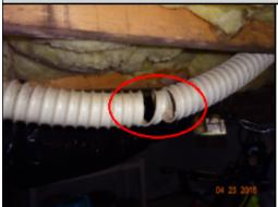
The bathroom vent ductwork is broken exiting conditioned air into the crawl space. A licensed general contractor or general repair specialist should be consulted for further evaluation to make sure the duct is proper installed and to make necessary repairs.
