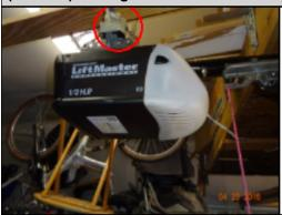
The garage door needs adjustment and repair. The electronic eyes are set too high to function properly because they have been mounted on top of the door opener. A garage door installation company or a licensed general contractor should be consulted for evaluation and repair to ensure that the door operates safely and properly.
