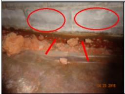
Additional Photograph: The efflorescence is circled and the mud has arrows. This a photograph of the moist areas that border the majority of the crawl space with the highest concentration by the deck. The white efflorescence on the brick wall is an indication of reoccurring moisture. This is evidenced throughout. The whole circled in the picture did not show evidence of deterioration. This most likely happened during construction and there is not a whole on the other side.
