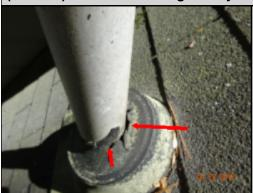
The two of vent boots located over the master bedroom that acts as a flashing to prevent water penetration around the plumbing vent pipe are split, cracked and leaking. A licensed roofing contractor should be consulted for evaluation and repair to ensure the weather-tightness of the roof covering system.
