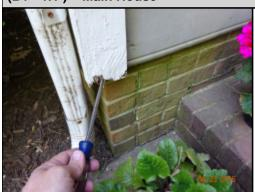
A siding installation company or general contractor should be consulted to evaluate and repair the trim to ensure the integrity of the cladding system. This is located by the front step.
