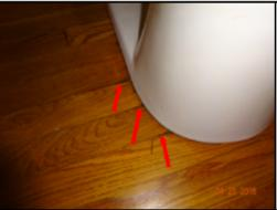
The toilet is leaking. The wax ring needs to be repaired to secure the toilet and ensure sanitary conditions. Notice the discolored lines in the wood flooring. The sub floor in the crawl space was not rotted on the underside. A licensed plumbing contractor should be consulted for complete evaluation and of the waste line systems to determine the general condition of the system and to make necessary repairs.
