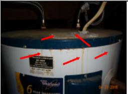
The water heating unit for this home is over ten years old and was found to be in poor condition. The unit has heavy corrosion of the casing and supply line connections. A licensed plumbing contractor should be consulted to evaluate the system and repair/ replace as needed to ensure safe and reliable hot water supply. The leak was not present at the time of inspection. Owner disclosure is suggested regarding any repairs.
