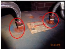
Additional Photograph: This is a photograph of the corrosion on the water heater.
