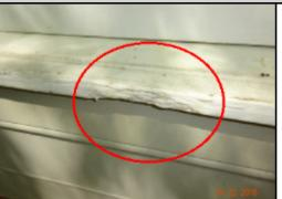
The dining room window(s) has/ have soft and decayed wood in the sill area. Decay in the windows can result in leaking and water penetration and should be repaired as soon as possible. All windows should be inspected for similar damage as repairs are made. A licensed general contractor should be consulted to evaluate the extent of the damage and make necessary repairs.
