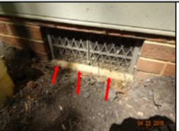
The grading around the foundation of the home is too high. Incorrect clearance can result in water penetration, drainage, and conditions inducive of insects and decay. A licensed general contractor should be consulted to evaluate and correct the grading as needed for proper clearance and drainage.
