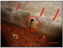
Additional Photograph: This a photograph of the moist areas that border the majority of the crawl space with the highest concentration by the deck. The white efflorescence on the brick wall is an indication of reoccurring moisture. This is evidenced throughout. The whole circled in the picture did not show evidence of deterioration. This most likely happened during construction and there is not a whole on the other side.
