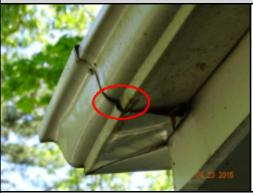
The gutter is bent and not sealed. Rain water leaks out onto the cement entry area. A licensed contractor should be contacted for repair.
