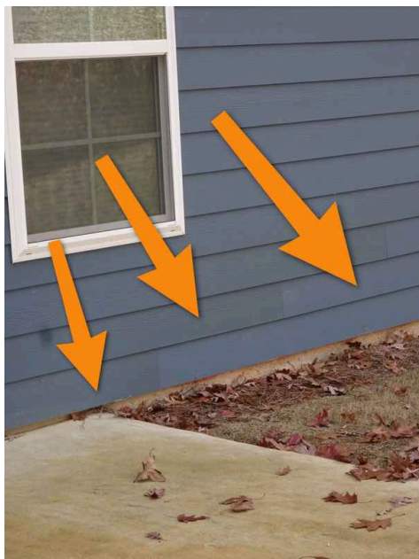
The siding is two different colors in this area.
