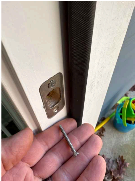
These light duty screws are half the length and half the diameter of the proper screws.
