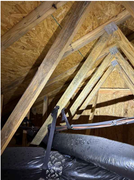
Microbial growth was also found in the small attic space off the right rear bedroom.
