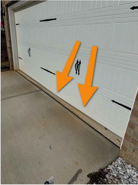
See description for this finding, the panel curves out here.
