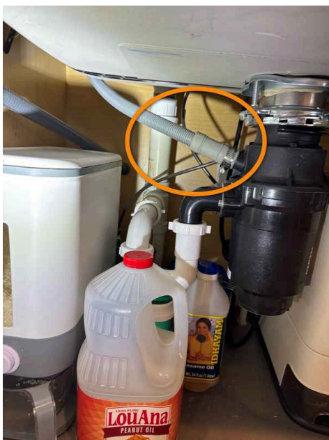
The plumbing lines for sink rattle when the water is turned on and off. The skin cause leaks.
