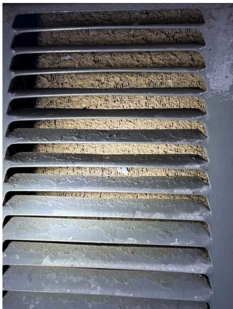
The coil is significantly dirty.
