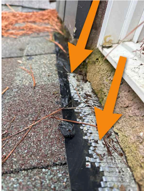
The flashing across the front middle of the home is bent up at the end. This direct water toward the home.
