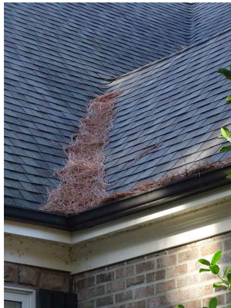
See description for this finding.
